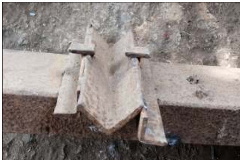
Fig. 8 Developed jig for bending plates
