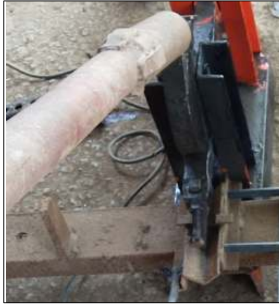
Fig. 9 Set of jig & fixture for manufacturing frame
