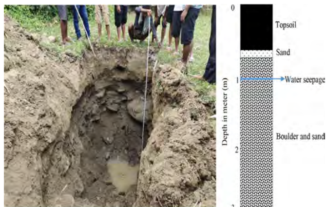
Fig. 9: Excavation of Pit (P1) at Dumrighari (left) and detail lithology of the pit (right) (GPS: 27.118732N, 85.543326E)
