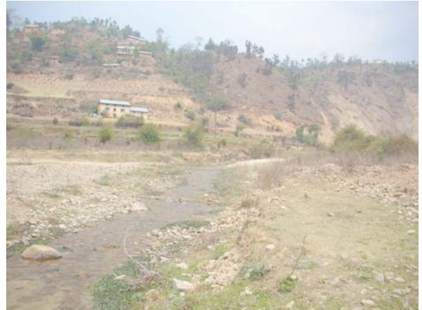
Fig. 8 Downstream view of the segment 4 of the Nakhu River at Nallu area
